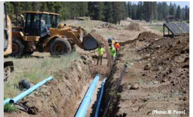
Intensive upgrades include a domestic water line installation heading up the Lower Galena Trail.
